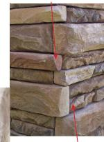
Alternate corner and flat stones so as to not create a vertical stone line
